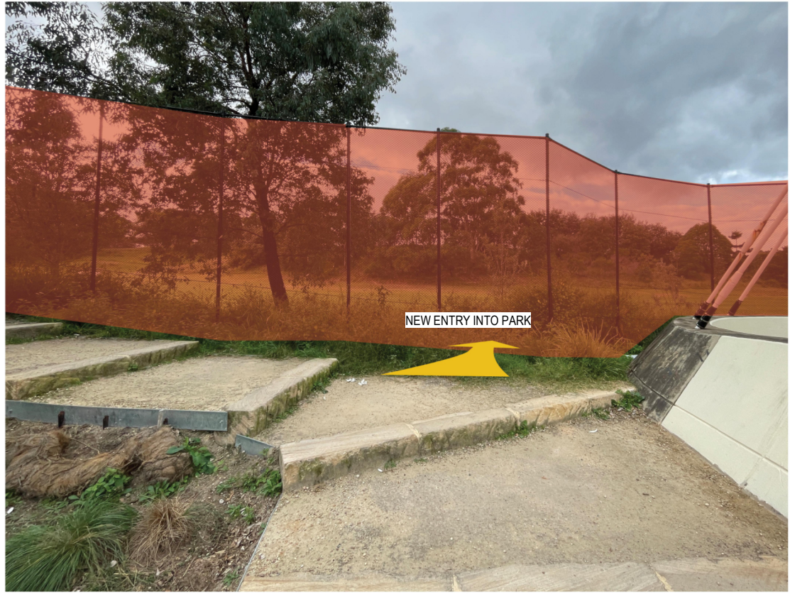
4. RESHCS BRIDGE ENTRY VIEW 2
