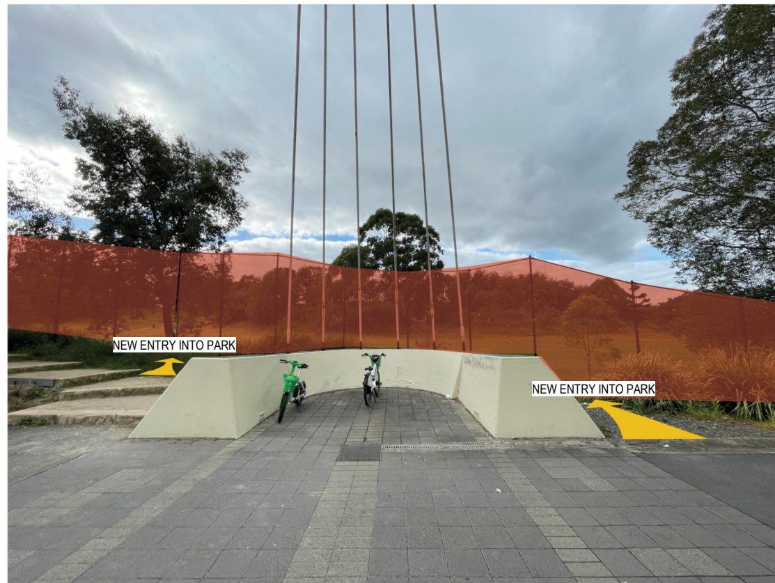
3. RESHCS BRIDGE ENTRY VIEW 1
